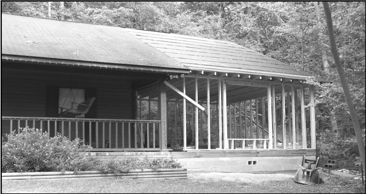
The addition onto Charles' home, during the early stages of construction.
